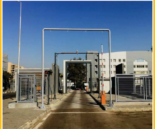
System installed in Egypt
